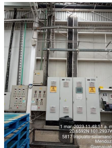
Photo 18: Main electrical panel
